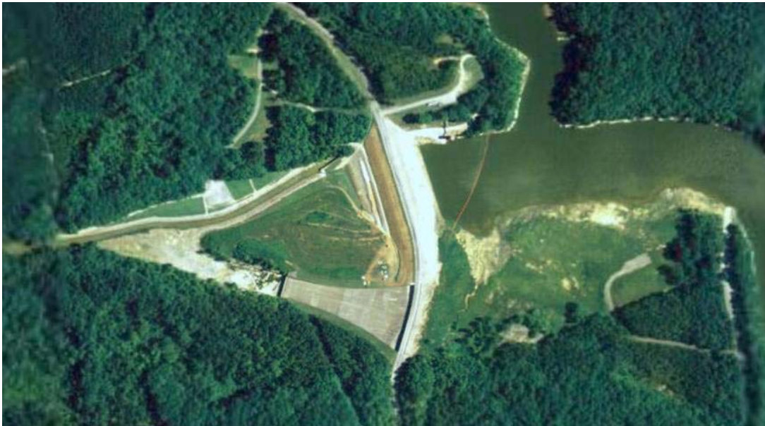
Figure 2. Photograph of Bear Creek Dam, Spillway and Outlet Works
