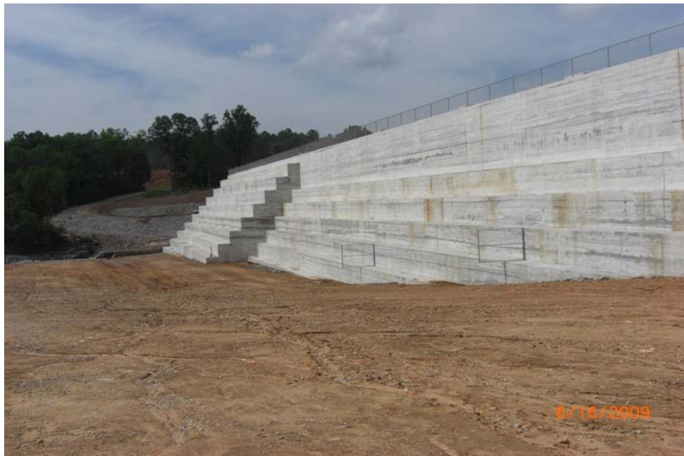
Figure 13. Photo of Downstream Face of Completed Berm
