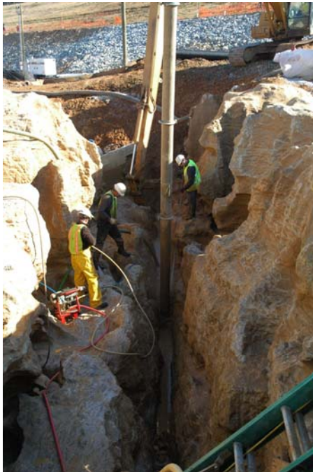
Figure 6. Excavation of Karst Feature along N30E Joint
